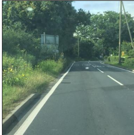
Photo 1: Southbound approach to bend at junction between Lower Burnham Road and Fambridge Road showing back of existing damaged map sign.
