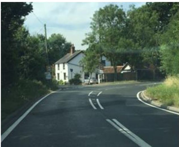
Photo 2 & 3: Southbound entry to bend and junction with Fambridge Road showing lack of chevron signing and the temporary fencing following a recent collision.
